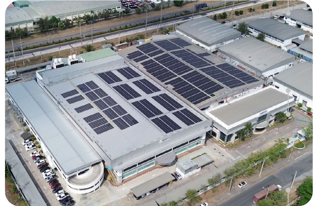
Solar panel system at our Thailand facility.
