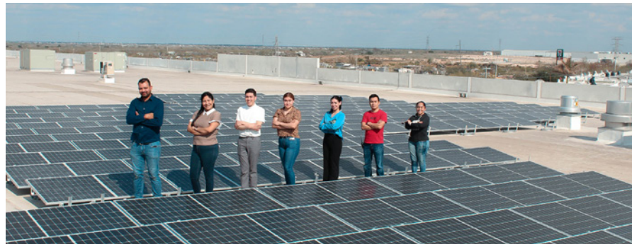
Top picture shows our solar installation in Thailand. Bottom picture shows our installation in Mexico.
